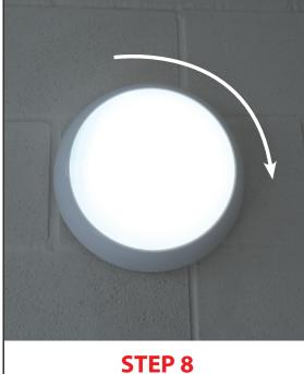
Twist lock diffuser in place
