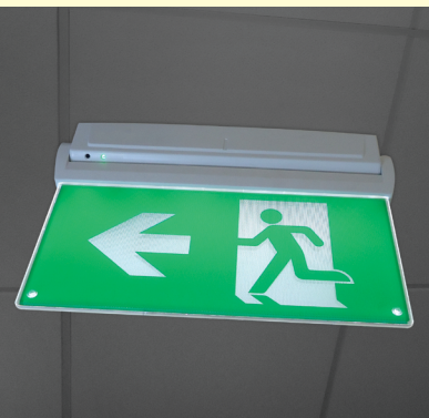
3) Push the EXITMMO into the EXITREC until it is secured in place
