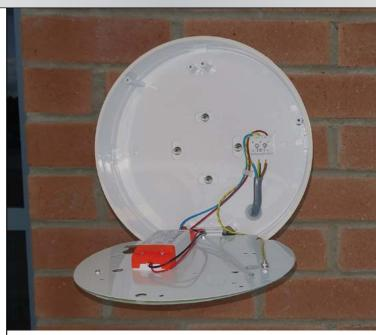
STEP 3 Fix base to mounting surface
