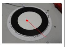
Lift out and remove Reflector assembly
